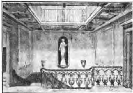
Staircase, 160 High Street, Hull.
